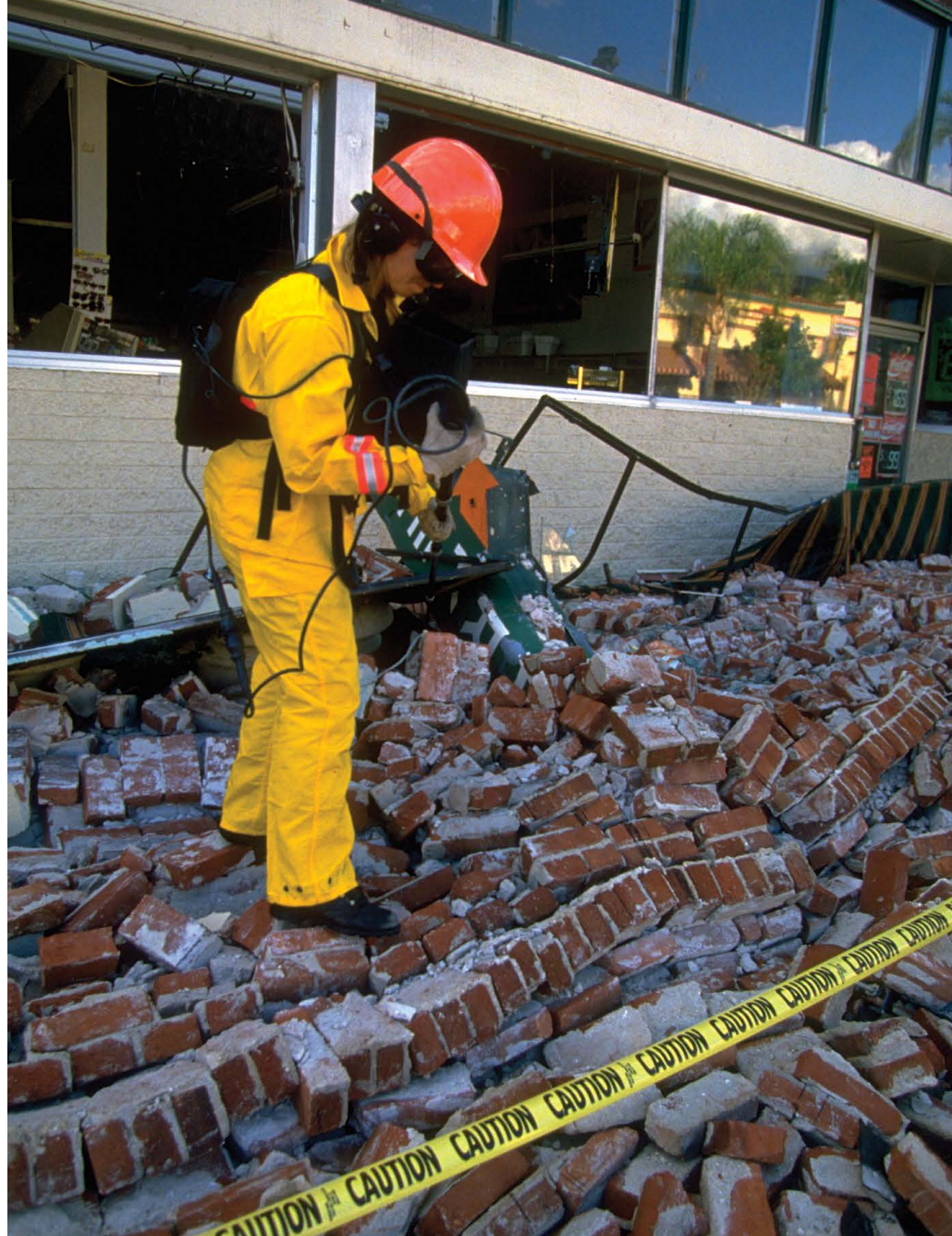
Shown here, failure of an unreinforced masonry building in the 1994 Northridge, Calif., USA, earthquake. (Photo courtesy of FEMA)
